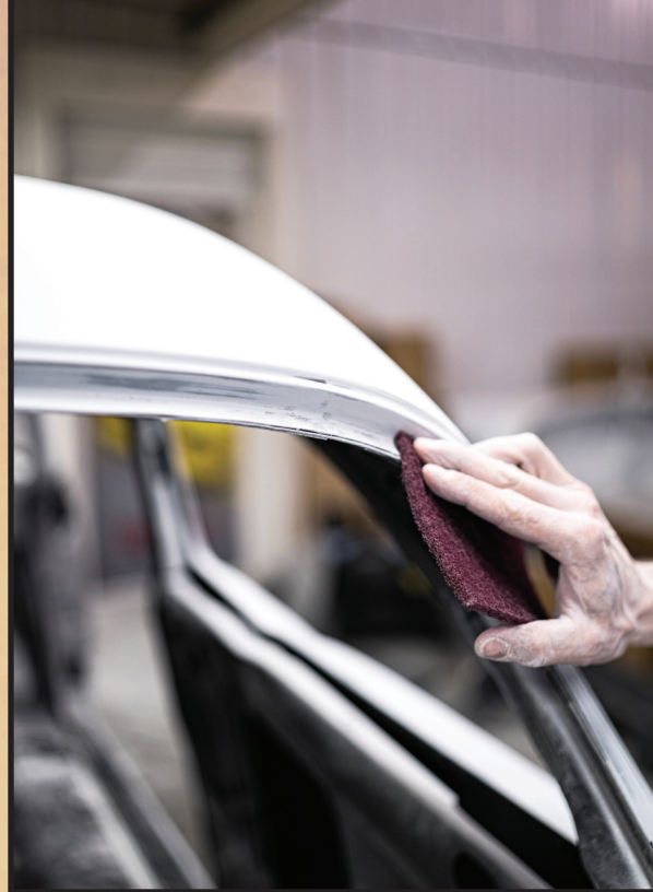
Scuffing: not everyone's favorite job, but a necessity. Use these scuff pads to get all the tough places sandpaper cannot reach, such as spot weld indentions and tight corners.
